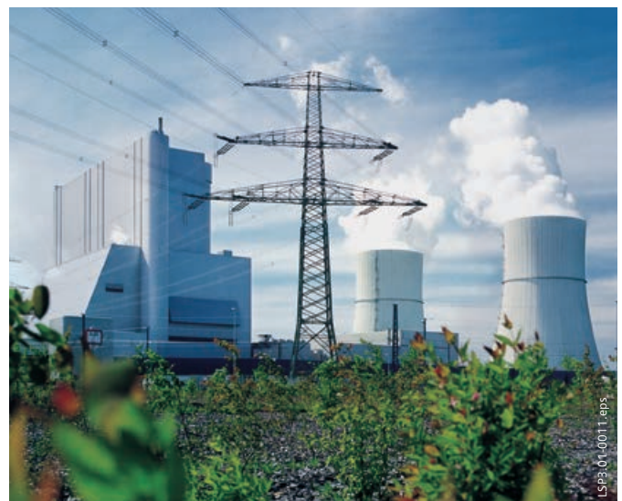
Fig. 1/14 SIPROTEC 4 application in power stations
